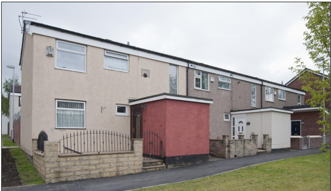
Crossley Estate houses before solid wall works started
