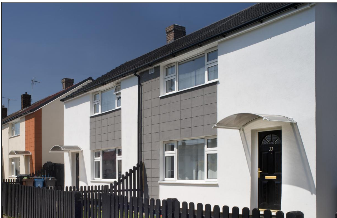
Holts estate homes after solid wall insulation works complete
