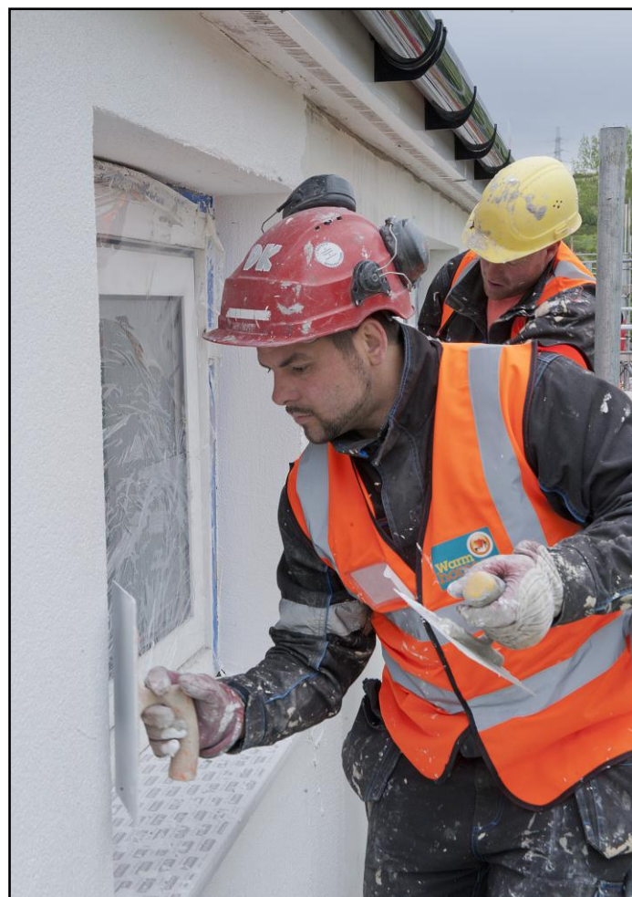
External wall insulation being applied to Holts
