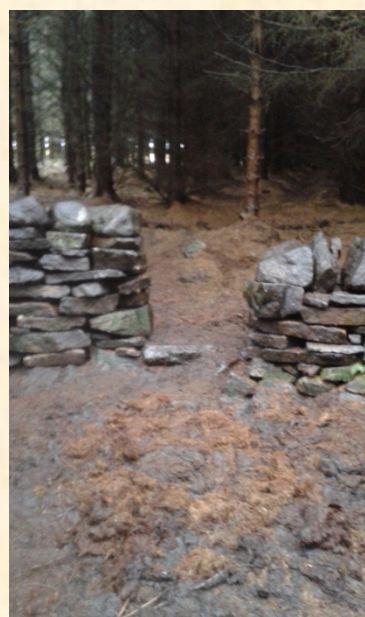
Dry Stone Walling Repairs
