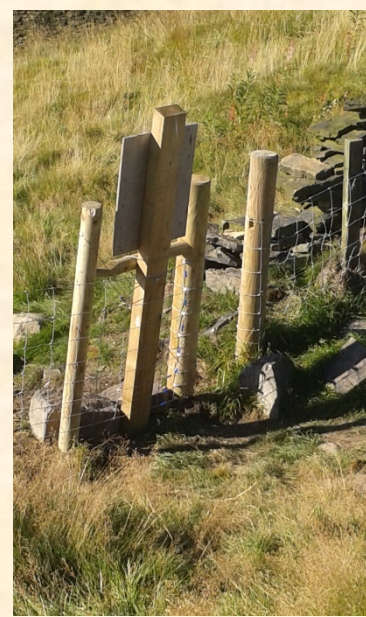
New & Repair Fencing
